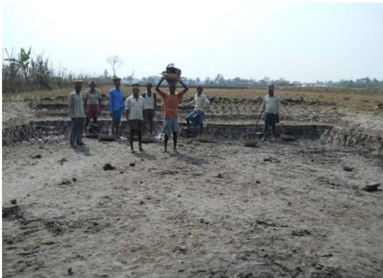
Plate 78– WHS construction in Sutahata, 22° 7'28.13"N 88° 9'34.75"E, Purba Medinipur
